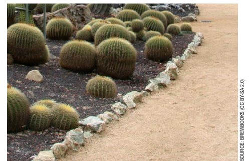
FIG. II.E.3: AGGREGATE EDGE This aggregate path is retained at the edge by a row of cobbles
