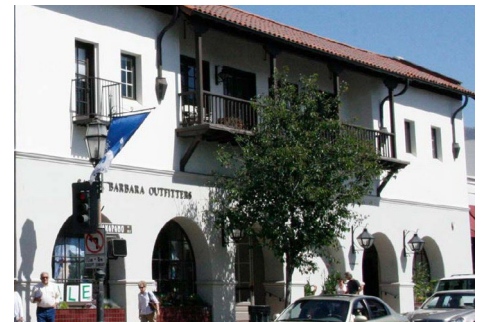
FIG. III.C.3: FLOOR LEVEL ARTICULATION This mixed-use building differentiates the ground floor with large gallery openings and a cornice.
