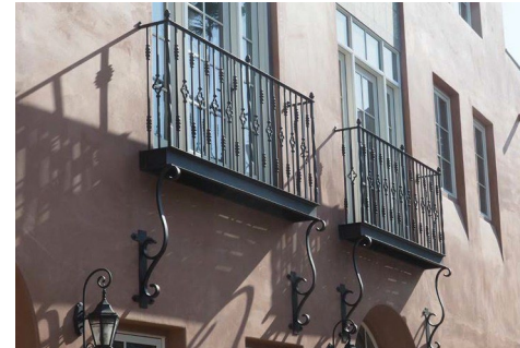
FIG. III.E.1: BALCONIES Wrought-iron Juliet balconies with supporting brackets on a traditional style building.
