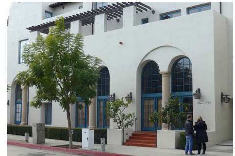
FIG. III.E.9: RECESSED DOORS Ground floor commercial entrances are recessed inside arches at this mixed-use project.
