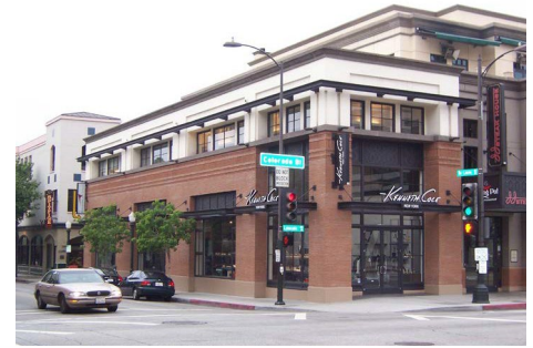
FIG. III.C.1: UPPER-STORY STEPBACKS The fourth story of this building steps back to respect the prevailing height of existing buildings on this street.
