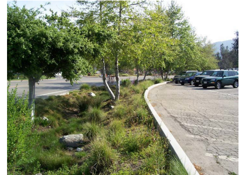
FIG. II.A.2: LANDSCAPED PARKING The planted area between parking rows is designed as a sustainable bioswale, which absorbs water run-off.
