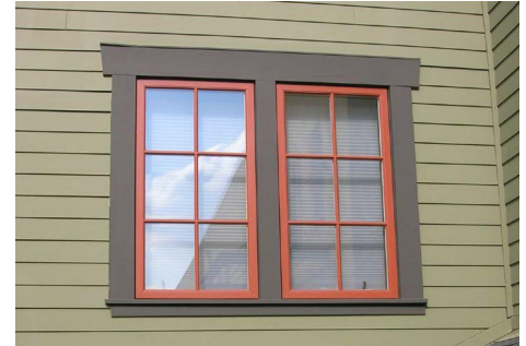
FIG. III.E.8: WINDOW TRIM This Craftsman style window trim includes head casing on the top that is wider than the jamb casing on the sides.
